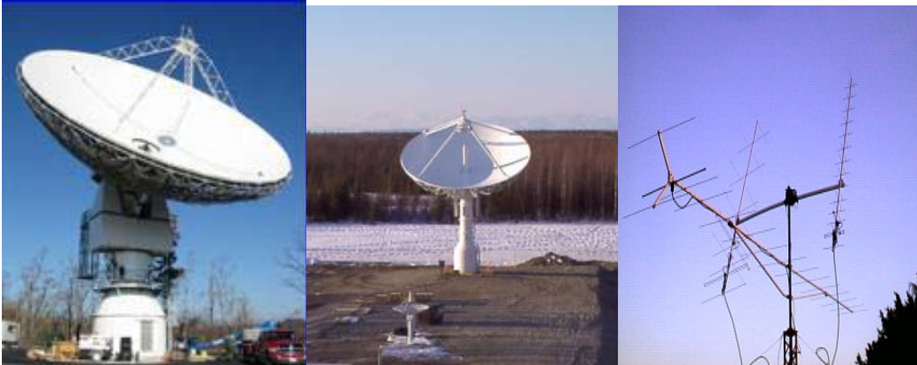
Figure 9. S-Band and UHF/VHF Antennas in RAMPART Ground Station Network
